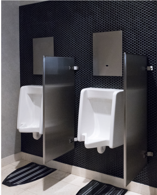
Water-conserving urinals operate in the range of 0.125 gpf (ultra-high efficiency) to 0.5 gpf (high efficiency).
